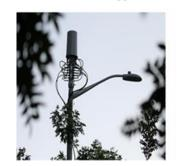
*Note:* Small-cell transmitter on a streetlight in Providence, Rhode Island. *Source:* The Providence Journal (Glenn Osmundson, 2017<sub>[81]</sub>).
